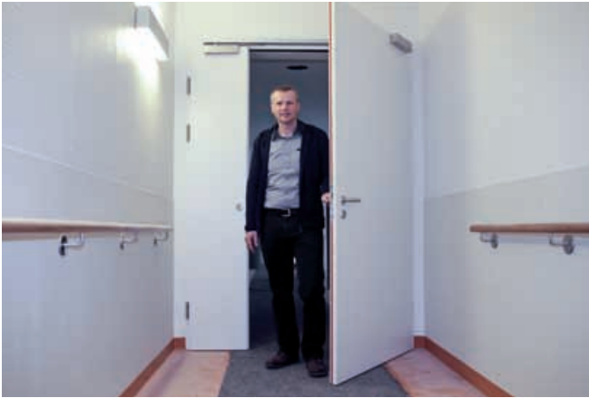
▲ Reinhard Spendlhofer demonstrates one of the doors in the IWP Liebhartstal, which is fitted with the SR-EF-1S slide rail from ECO. Photo: Alfred Pany
